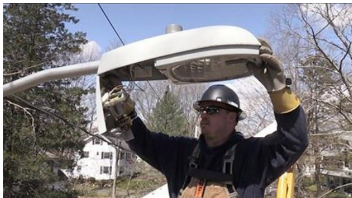
Wellesley Municipal Light Plant Line worker installing energy efficient LED Lighting.
