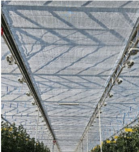
High-efficiency heat curtains at the Backyard Farms greenhouse in Madison, Maine.
